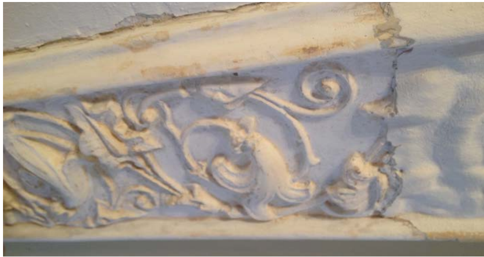
Figure 2.18. The delicate original shapes are not recognizable through the many coats of paint on the right. Photograph by Liv Berntsson.
