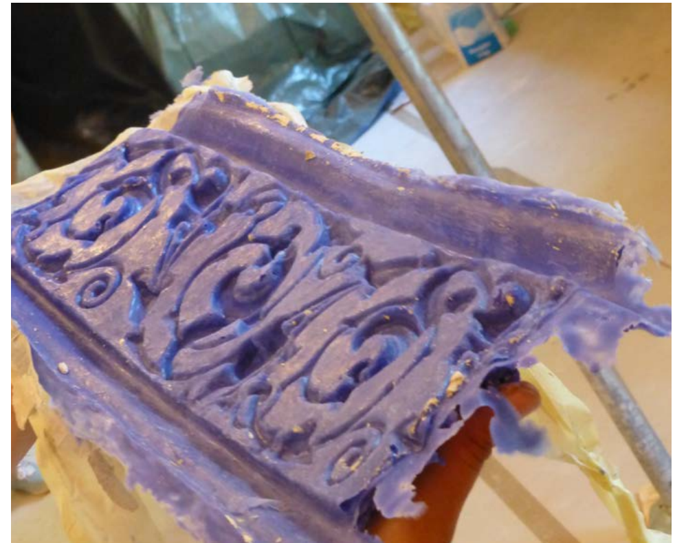
Figure 2.24. The silicone mould is ready to be used. Photograph by Kirsti Horn.
