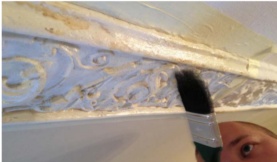
Figure 2.19. The original was touched up with gypsum plaster, sanded and brushed clean to give a perfect mould. Photograph by Liv Berntsson.
