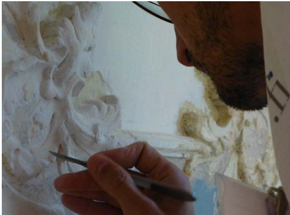
Figure 2.34. It took a whole week to clean and repair one acanthus motif. Photograph by Kirsti Horn.
