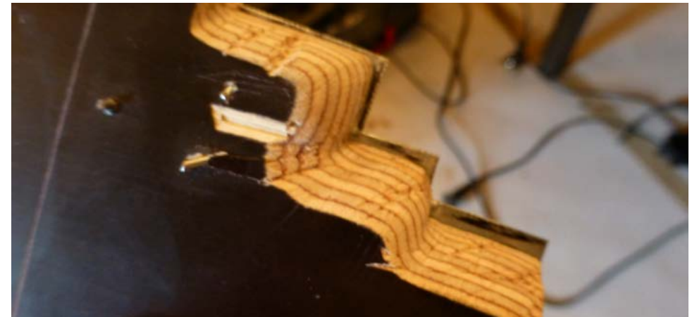
Figure 2.26. The documented moulding profile was transferred on metal sheeting and cut precisely in this shape. A piece of plywood was shaped accordingly and then attached to one side of the metal sheet. Photograph by Kirsti Horn.
