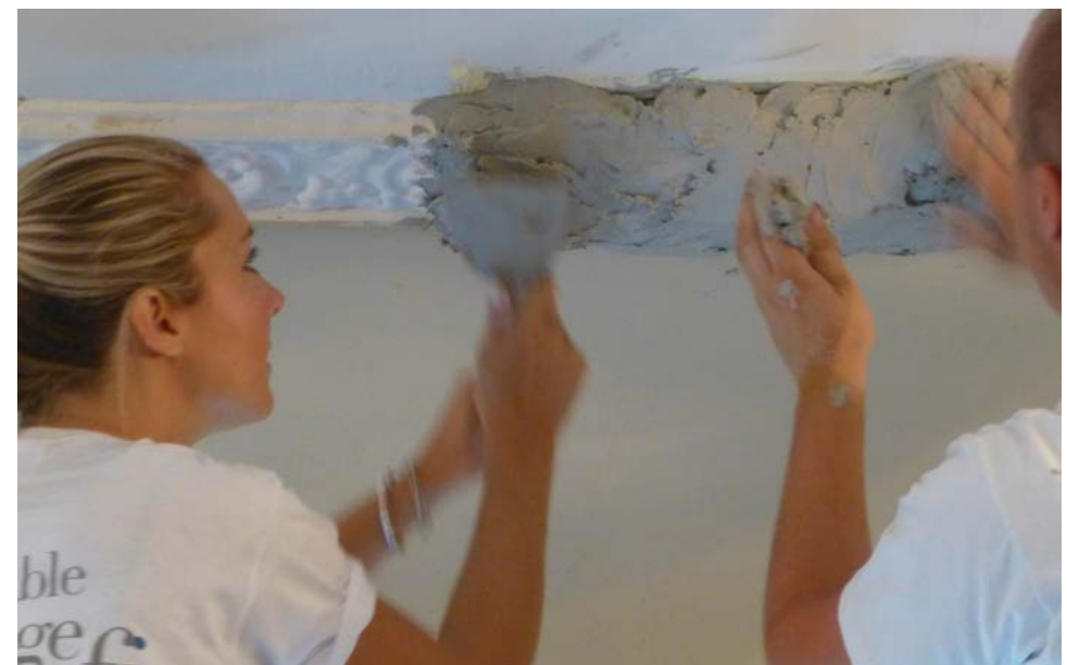
Figure 2.21. The silicone was covered with plaster and the whole package was left to dry. Photograph by Kirsti Horn.
