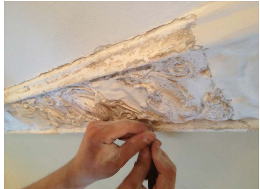
Figure 2.17. Working through many coats of paint. Photograph by Liv Berntsson.
