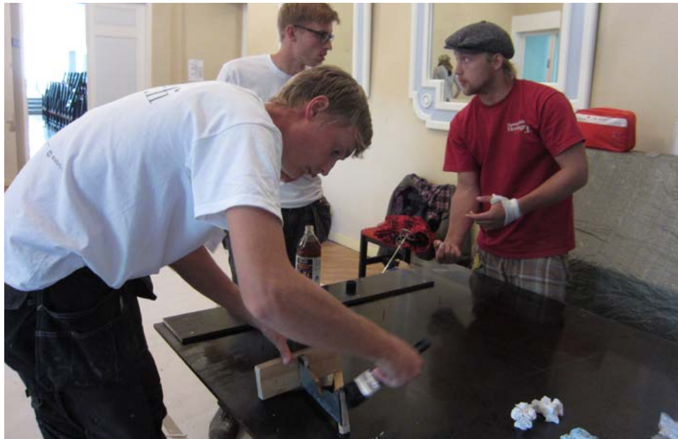
Figure 2.28. A wooden rail was attached along one side of the working table. The table and mould were oiled to start with. Photograph by Meelike Naris.
